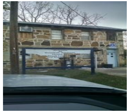
Front of Bldg.
